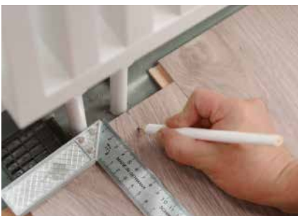
Door frame and radiator pipes
